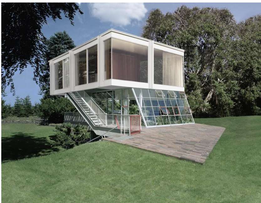
Fig. 5: Baukunst, House on a Hill , 2009
